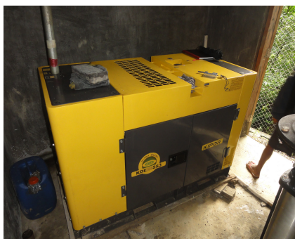
(b) Diesel generators supplying electrical power for high-lift pumping, Ethiopia (left) and Timor-Leste (right)
